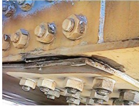
Figure 10: Corrosion – Case 1.
