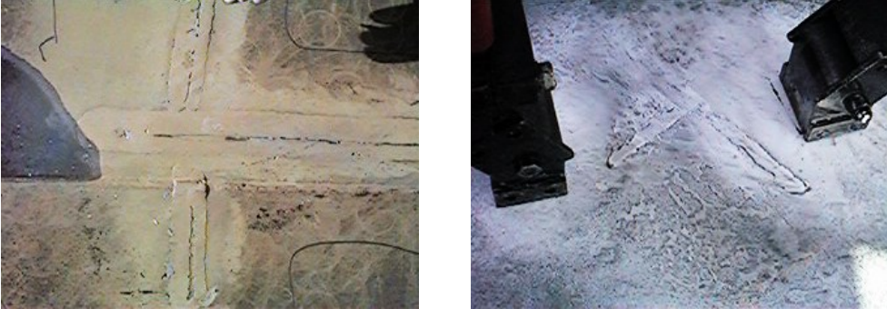
Figure 5: Fabrication defects – Case 2, two different examples.
