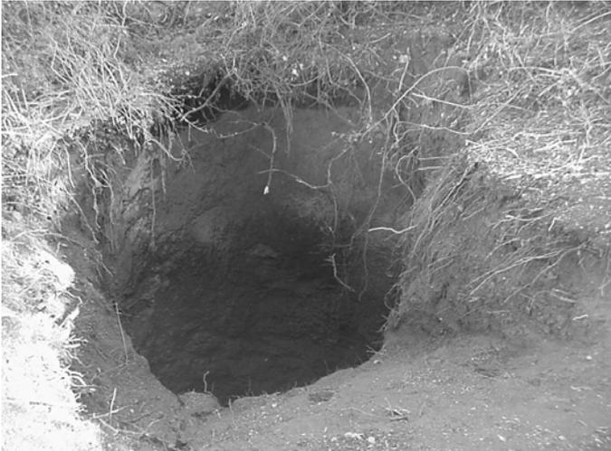
Figure 13: Collapse of the filling of a karstic chimney crossed by Dodoni Tunnel. The collapse outcropped on the surface about 100 m. over the tunnel.
