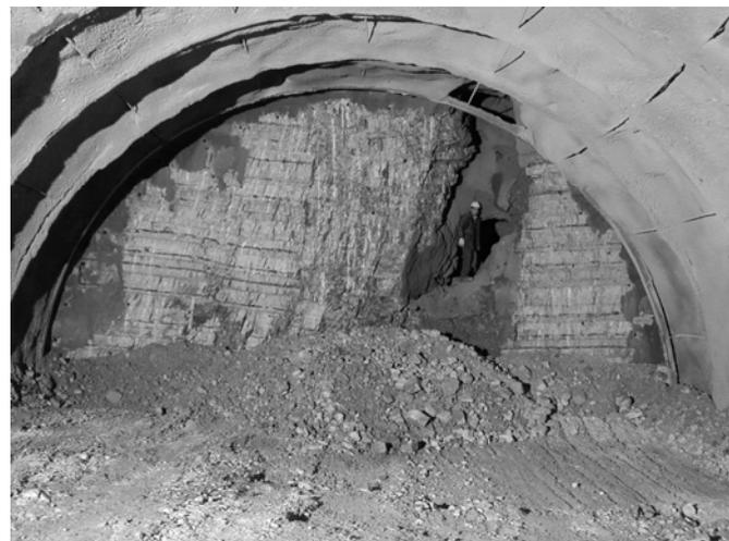
Figure 12: Typical appearance of a small karstic void partially filled with clay and silt; Dodoni tunnel, northwestern Greece, 2000.
