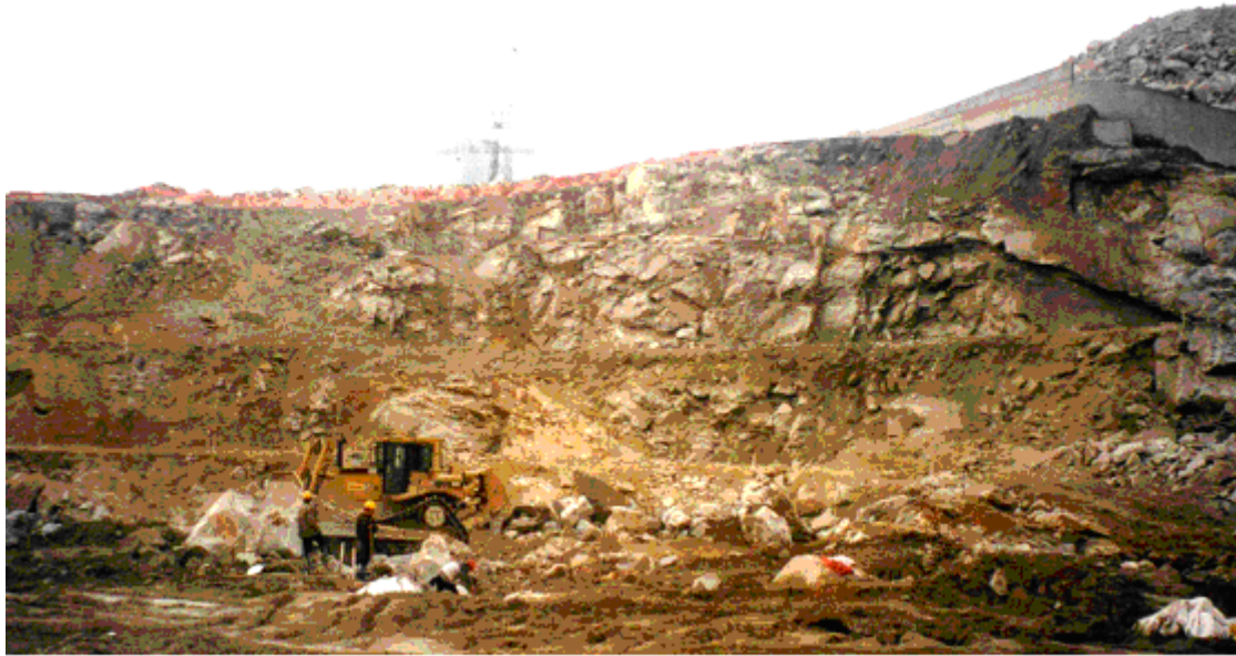
Figure 4: Appearance of Oporto granite in the face of an excavation for the new football stadium. Fracturing of the rock mass and heterogeneity of weathering is obvious
