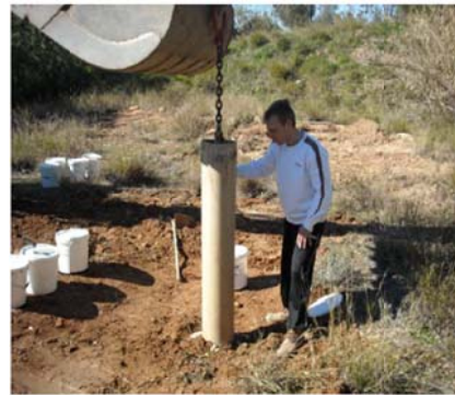
Figure 2. Installation of grounding systems at NTUA Campus.
