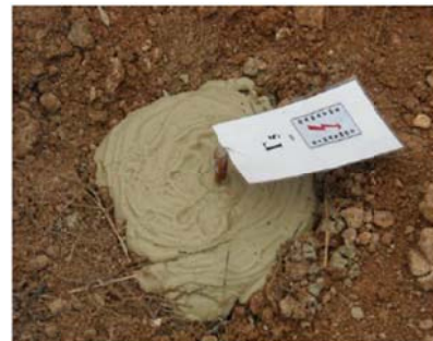
Figure 3. Installation of grounding rod with ground enhancing compound.
