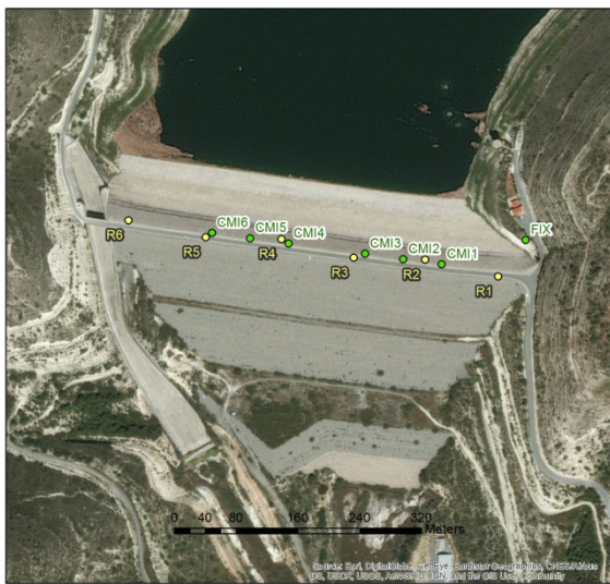
Figure 2: Instrumentation on the dam crest
