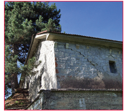
Picture 4: Damage caused by structural deformation
