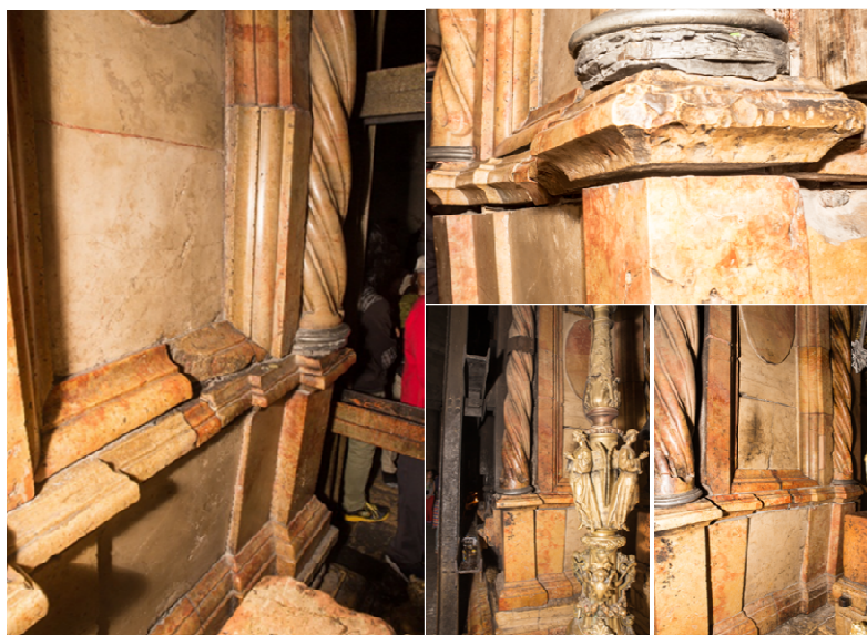
Figure 9 External facades deformations
