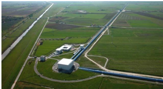
Aerial view of the site of the Virgo (near Pisa, Italy) experiment showing the central building, the Mode-Cleaner building, the full 3 km-long west arm and the beginning of the north arm (on the right).
