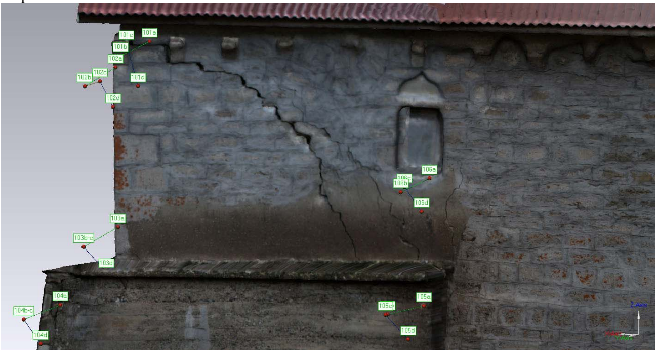
Figure 10: Part of the external northern façade
