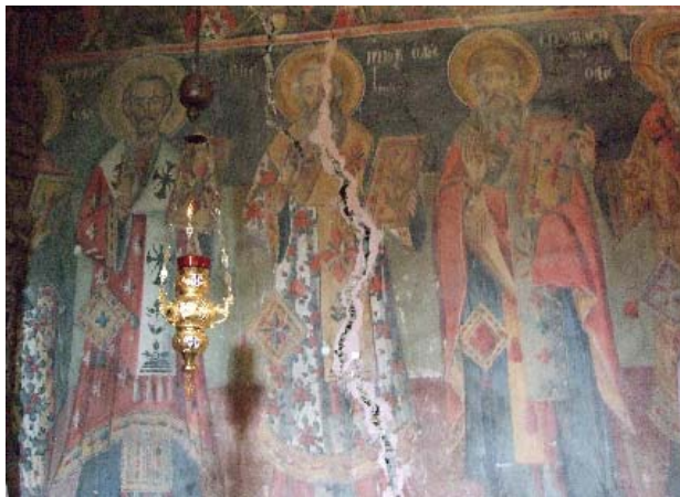
Figure 2: Typical examples of damage caused by structural deformation in the interior (left) and the exterior (right) of the church of Megali Panayia in Samarina
