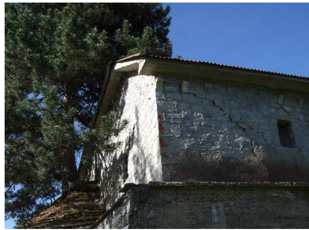
Figure 2: Typical examples of damage caused by structural deformation in the interior (left) and the exterior (right) of the church of Megali Panayia in Samarina
