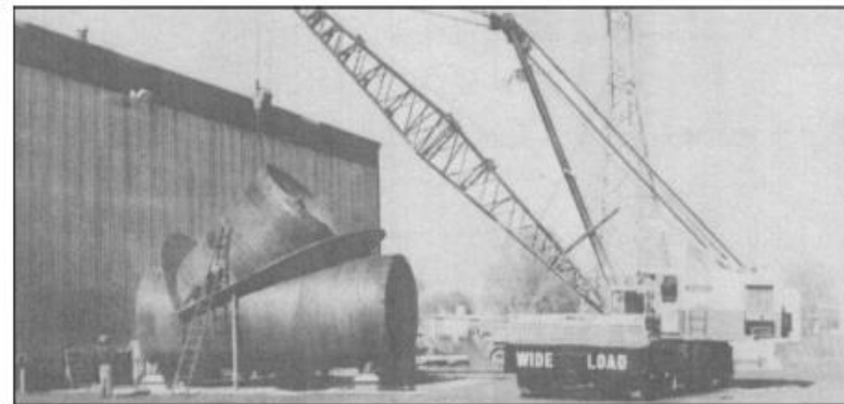
This 126-in. \times 126-in., 45° wye section has two plates.
