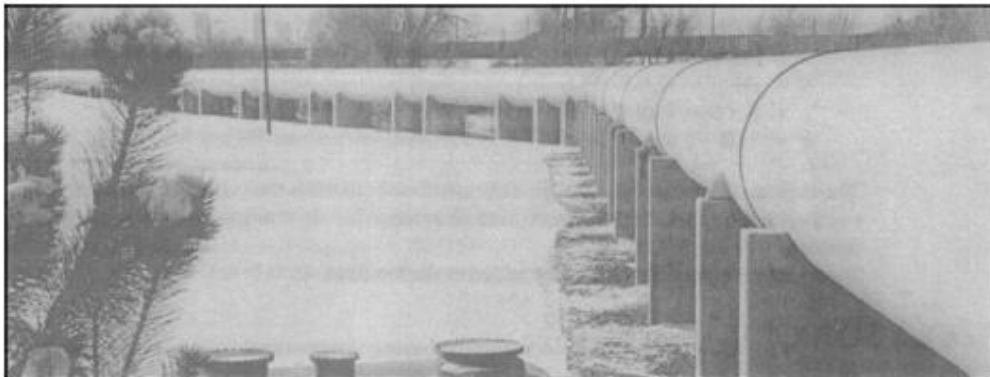
Figure 7-2 Saddle supports for 78-in. pipe
