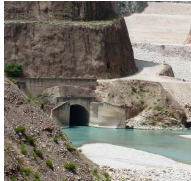
Entrance & outlet of diversion tunnel during construction of Hilarion dam
