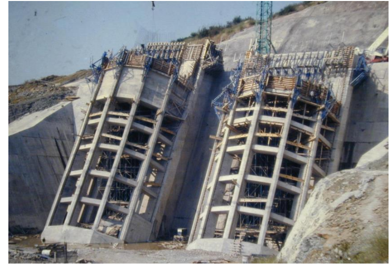
Stratos dam: inclined intakes under construction
