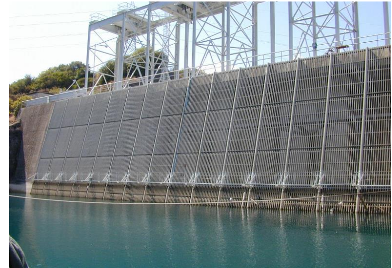
Kastraki dam: trash racks and gates
