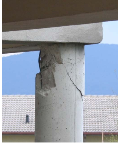
Figure 7.10. Shear failure of: (a) rectangular and (b) circular columns.
