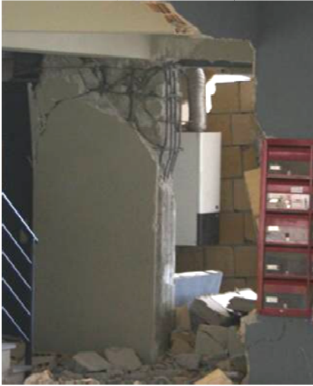
Figure 7.10. Shear failure of: (a) rectangular and (b) circular columns.
