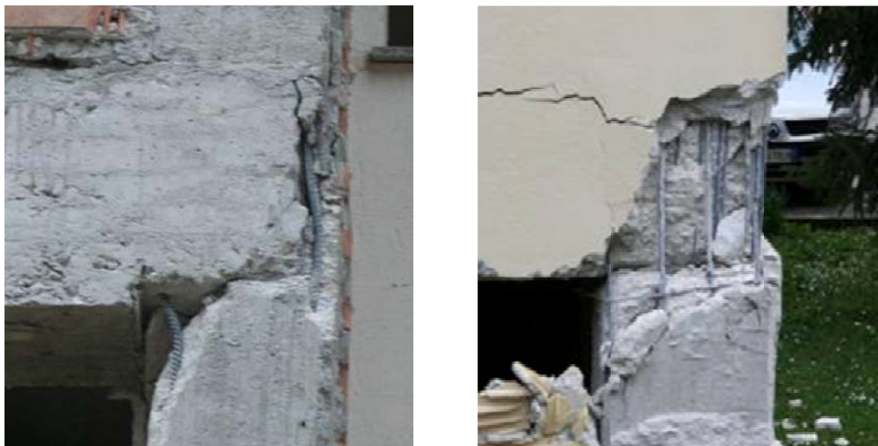
Figure 7.15. Failure mechanisms at joint – column interface surfaces
