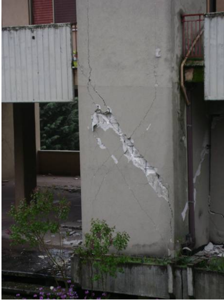
Figure 7.13. Failure in reinforced concrete walls.
