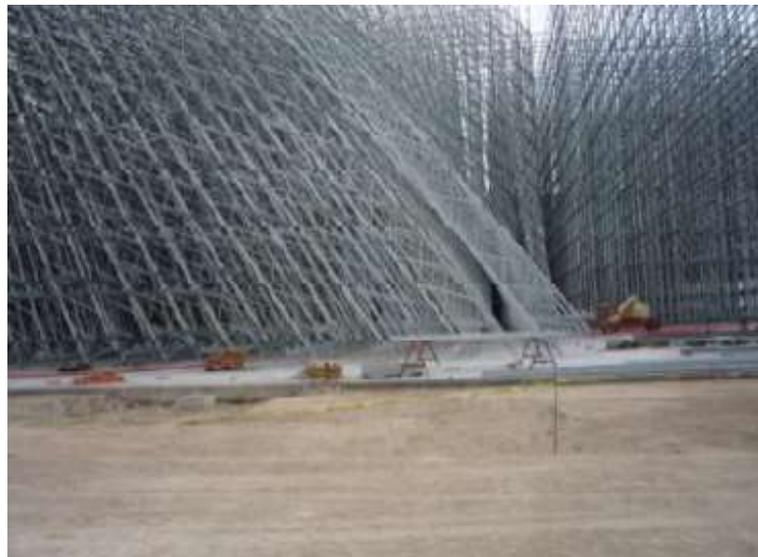
**Figure 1-7:** Premature collapse of an ARSW during construction phase<sup>3</sup>
