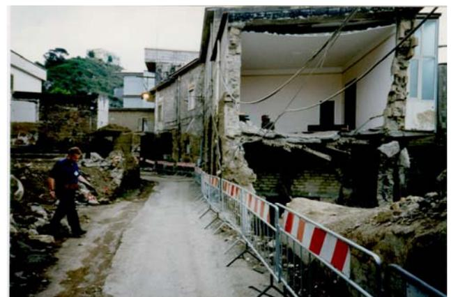
Figure 6a,b: (a) Masonry building impacted by debris flows; (b) Residual parts of masonry buildings
