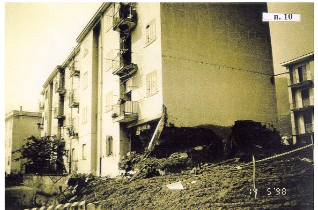
Figure 5a,b: R.C. structures: (a) Plastic collapse mechanism of columns; (b) Failure of corner column.
