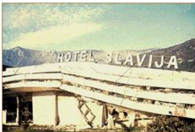
Figure 6. Damages caused by the earthquake on the 15 th of April 1979: a detail from “Slavija” hotel – Budva (source: Ministry of Interior and Public Administration)
