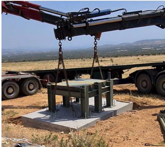
Figure 6-3: Installation of the prefabricated experimental setup in the pit
