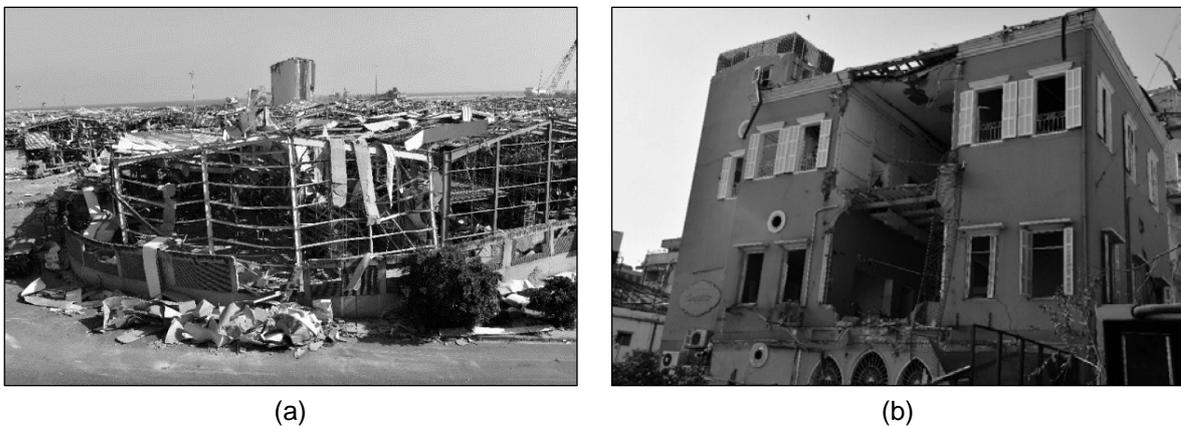
Figure 1-7: Failures in the Beirut explosion [reprinted from [Lekkas et al. \(2020\)](#)]: (a) Metal sheets; (b) Masonry walls
