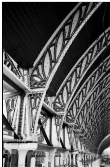
Figure 1-1: Curved cast iron in roof trusses (King and Brown, 2001).
