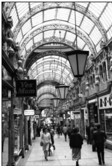
Figure 1-1: Curved cast iron in roof trusses (King and Brown, 2001).
