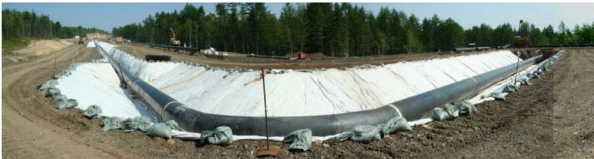
Figure 2-11: Construction of the dog-leg structure at the pipeline – fault crossing at Sakhalin (Besstrashnov and Strom 2011)
