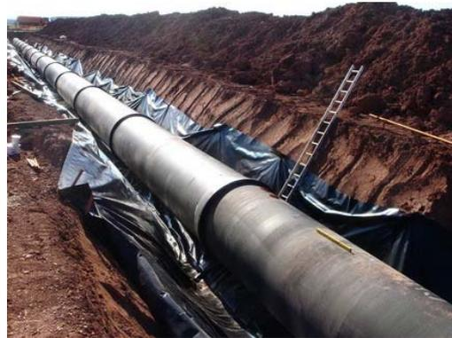
Figure 2-16: Construction of segmented pipe with ball joints (Xinxing Pipes International Development Co. Ltd. 2016)
