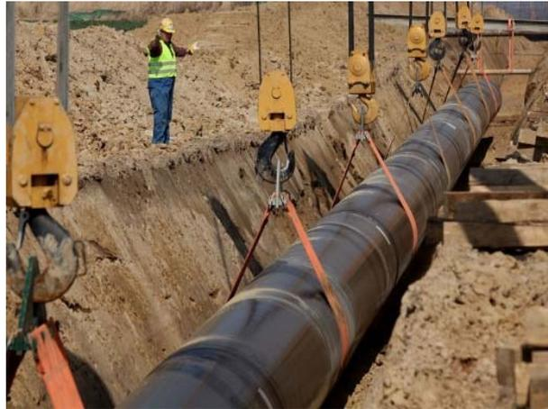
Figure 1-3: Buried pipeline construction ("ConstructionWeekOnline.com" 2016)
