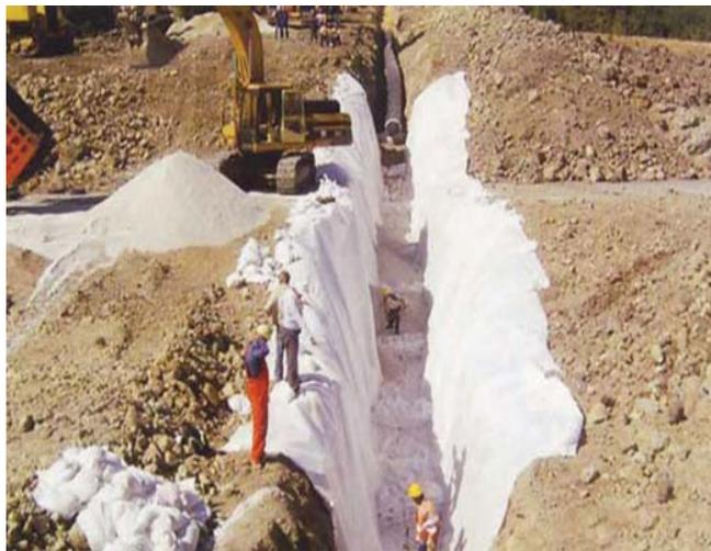
Figure 2-9: Pipeline wrapping with friction-reducing geotextile (Gantes and Bouckovalas 2013)
