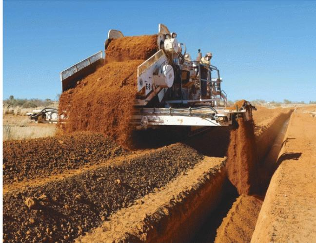
Figure 2-8: Trench backfilling with graded soil
