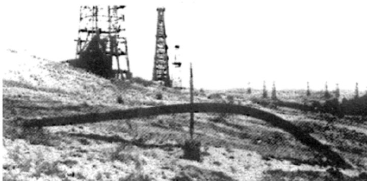
Figure 1-11: Upheaval buckling of onshore buried steel pipeline due to faulting (Yun and Kyriakides 1990)
